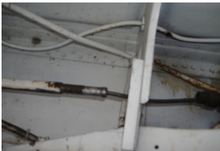
conduit jammed by crud
