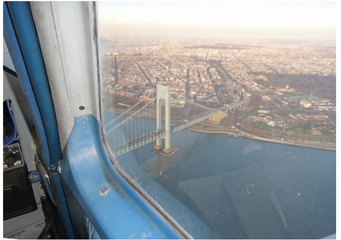
Verrazano Narrows Bridge
